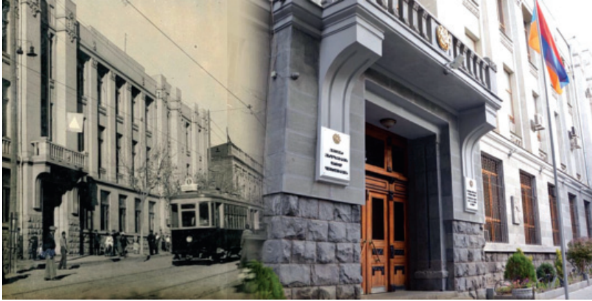
The building of the Prosecutor General's Office of the Republic of Armenia, built in 1936, designed by Baev. The building is included in the state list of immovable monuments of history and culture of Yerevan, Republic of Armenia
